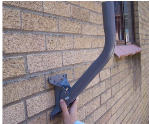
Figure 4-3 – Pole Assembly
